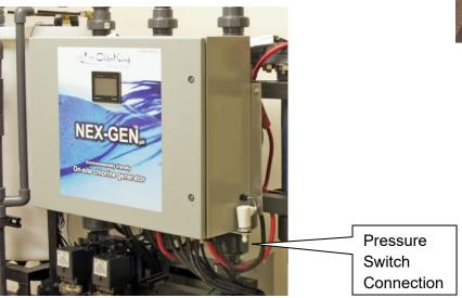
Connect the pressure switch to the return line with  $\frac{1}{4}$  tubing (not supplied) and the  $\frac{1}{4}$  inch valve supplied. The pressure connection should provide a minimum of 5 psi when the pool pump is on, and pressure should be less than 3 psi when the pool pumps are off. Contact ChlorKing for installations that do not meet these specifications.
