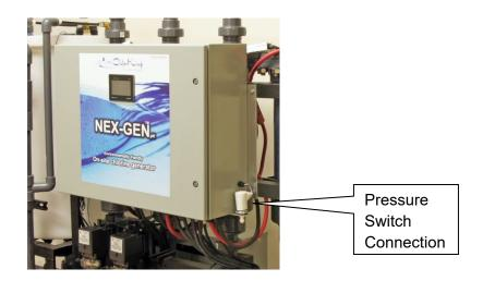
Connect the pressure switch to the return line with  $\frac{1}{4}$  tubing (not supplied) and the  $\frac{1}{4}$  inch valve supplied. The pressure connection should provide a minimum of 5 psi when the pool pump is on, and pressure should be less than 3 psi when the pool pumps are off. Contact ChlorKing for installations that do not meet these specifications.
